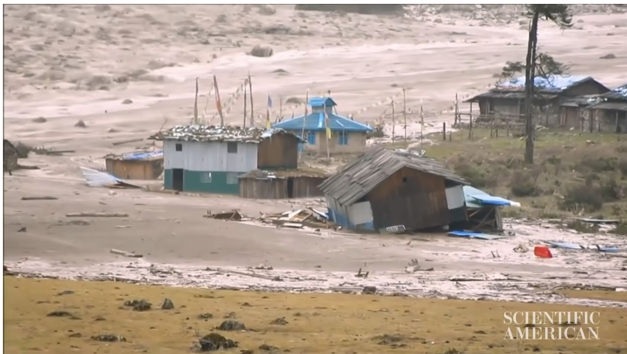
Figure 3. Damage to infrastructure from a GLOF experienced by downstream communities in Yangle Kharka, Sankhushabha District, Nepal in 2017 18 .
