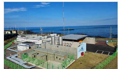
Hangwon Green Hydrogen Demonstration Complex, Jeju
