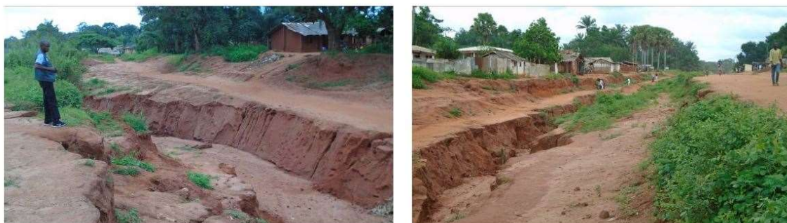
Photo 6: Erosion of a road in Berberati by run-off water, leading to its abandonment and the creation of another road. (TNC field mission, May 2018)
